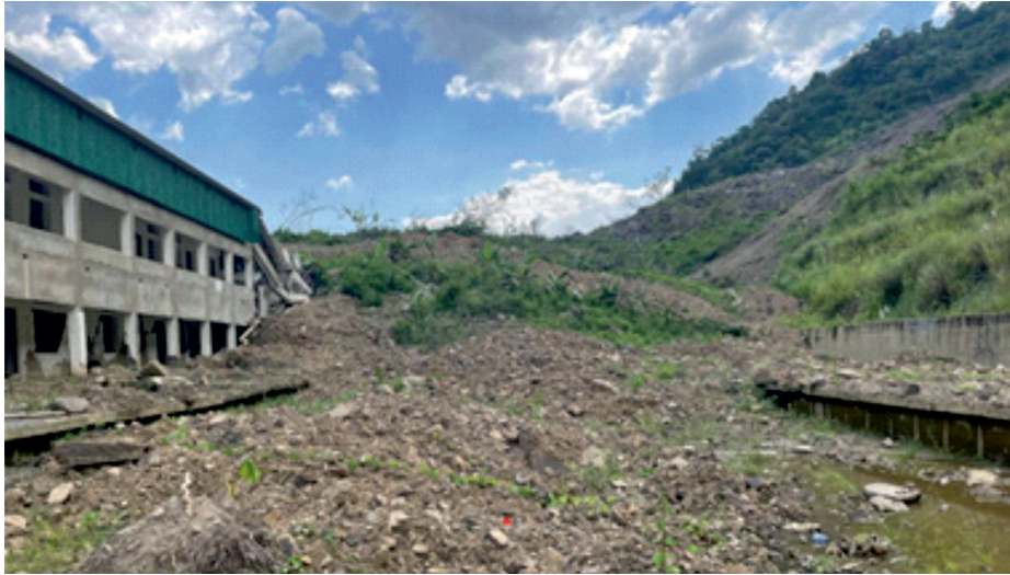
Fig - 68 : A railway station affected by the landslide
