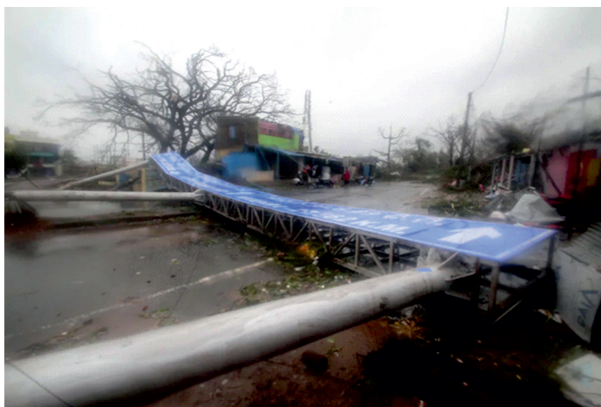
Fig - 4 : Damaged sign lies on a street in Puri
