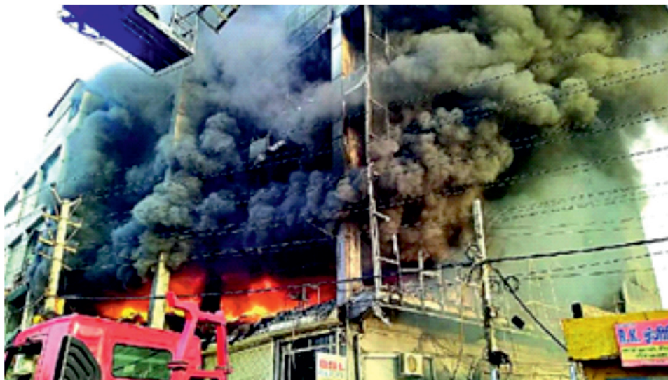
Fig - 83 : Fire at four-story commercial building
