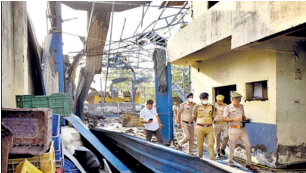
Fig - 64 : Investigation underway after an explosion inside a factory in Uttar Pradesh's Hapur
