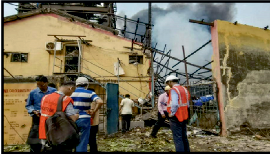
Fig - 98 : Firefighters at the spot after a fire broke out due to a boiler blast in a chemicals factory, at Dombivli, in Thane district, Maharashtra (PTI picture)
