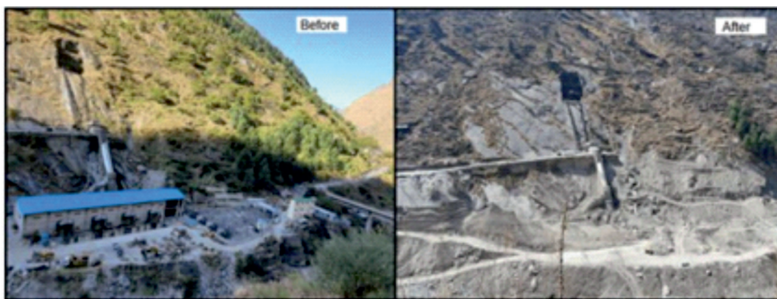
Fig - 50 : Before and after images of the Rishiganga HEP
