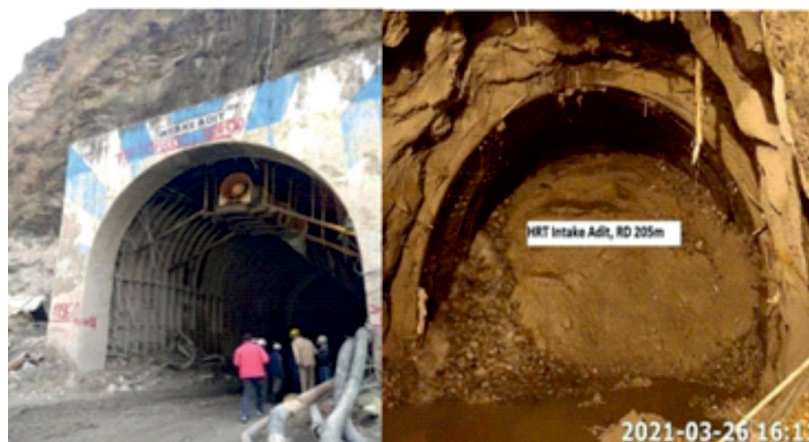
Fig - 53 : Outside of the intake Adit tunnel with HFL of 1801 m with submerged inside of the HRT intake adit
