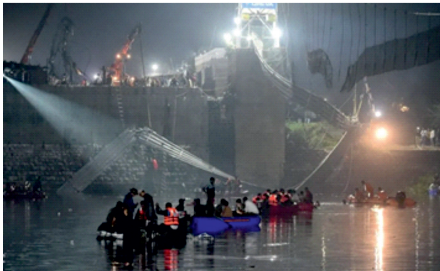
Fig - 79 : Morbi Bridge Collapse
