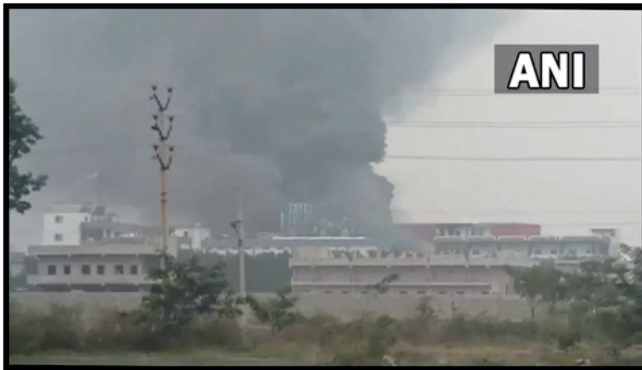
Fig - 99 : Tragic accident in Atchutapuram SEZ, reactor blast at Pharma Company
